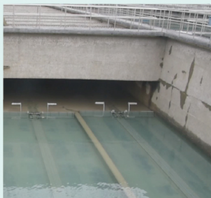
增設刮泥設備 進行即時排泥 Installation of sludge scraping equipment to perform real-time sludge discharge
