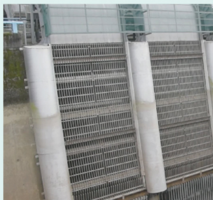
墊高耙污設備 確保取水穩定 Raised bar screen equipment ensures a stable water collecting
